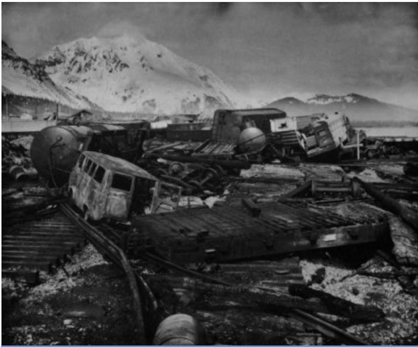
Damage in Seward
