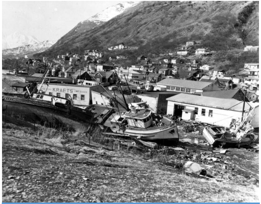
Damage in Kodiak
